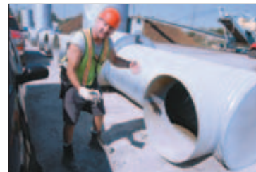
CONTROLLED ENVIRONMENT: Bernie Beechum, a Michigan Sugar pile operator, explains how steel pipes running through beet piles can deliver both warm and cold air to keep the temperature as constant as possible. Probes in the piles automatically turn the system on and off when needed.
