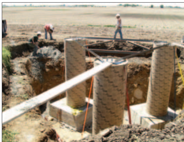
FARM POWER: Workers build the footings for the 120-foot-tall wind turbine that is being put up at the Hammer and Kavazanjian farm near Beaver Dam.
