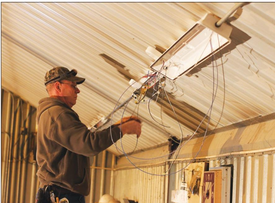
**DO IT RIGHT:** An electrician from Brown Electrical installs new light fixtures that are equipped with motion sensors to turn the lights on and off automatically at the ISU Armstrong Farm in southwest Iowa.
