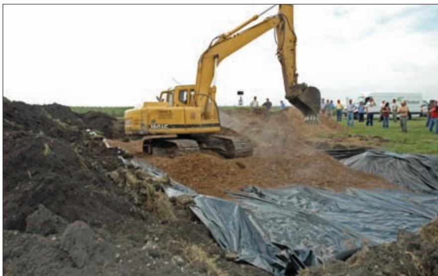
**ADD CHIPS:** Wood chips are spread over geotextile fabric at a bioreactor installation demonstration in Webster County. Wood chips serve as a carbon source to metabolize nitrate into gas.
