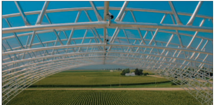
MORE TO STORE: Measuring 132 feet by 400 feet, Akron Services' new Brimfield hoop structure will store a million bushels of corn this fall.
