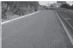
Pervious Pavement Installation
