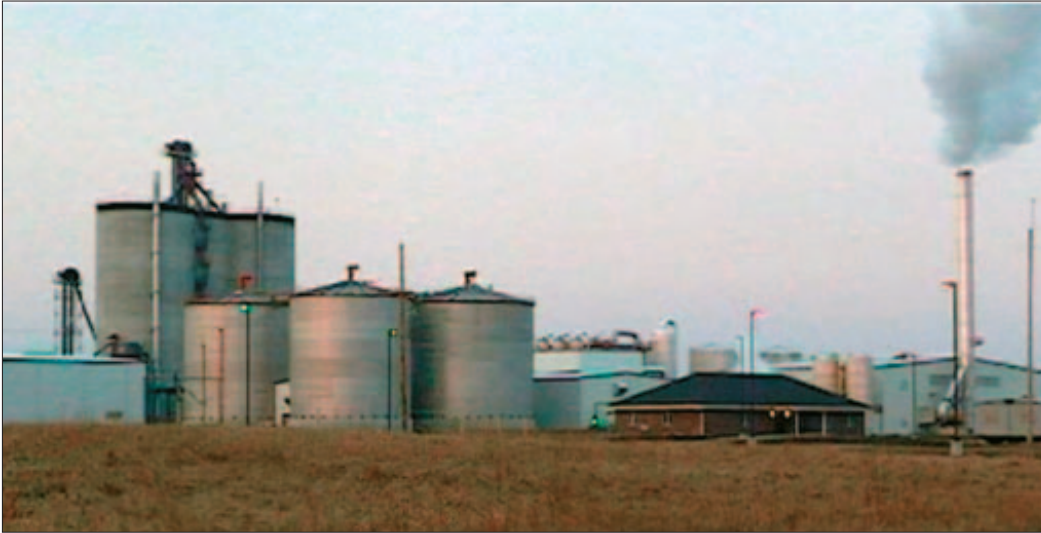
THE MID-MISSOURI Energy plant, a farmer-owned cooperative in Malta Bend, produces 40 million gallons of ethanol every year.
