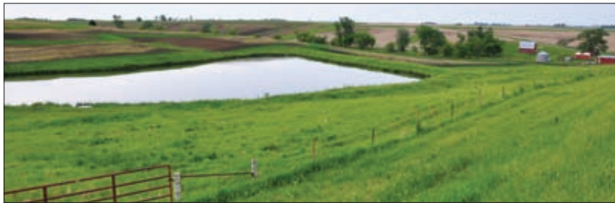
POND PRICES: A detailed, accurate cost estimate to build ponds like this one can be made in the NRCS office in less than 10 minutes using new computer software and LiDAR elevation data.
