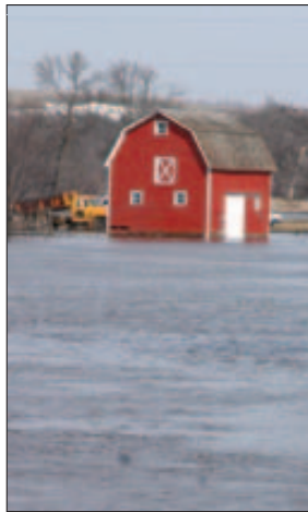
FLOATING? Water surrounds a red barn on a farmstead south of Valley City, N.D.
